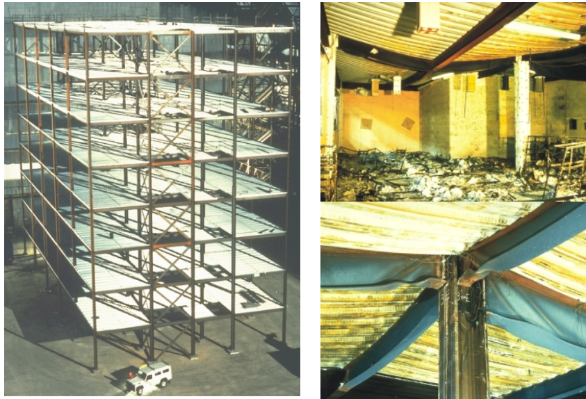
Figure 1: Cardington test building (left) Structure following the test (right)
