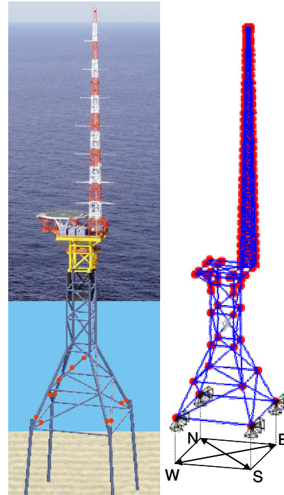
Figure 3: Research platform FINO 1 (photograph taken from [6]). a) Locations of strain gages. b) Numerical model and orientation with respect to nautical North
