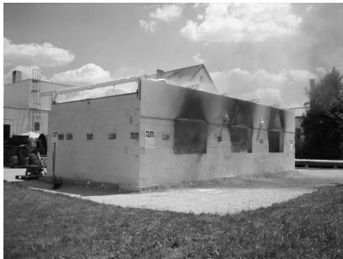
Fig. 1 First Munich fire test
