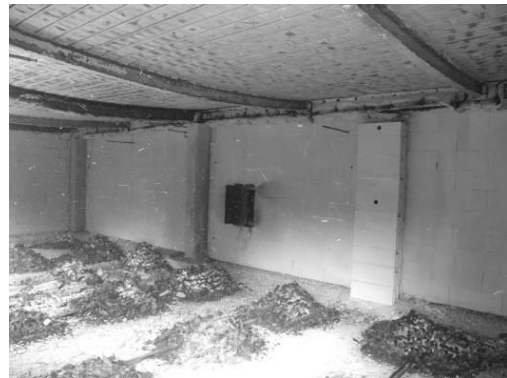
Fig. 2 Second Munich fire test
